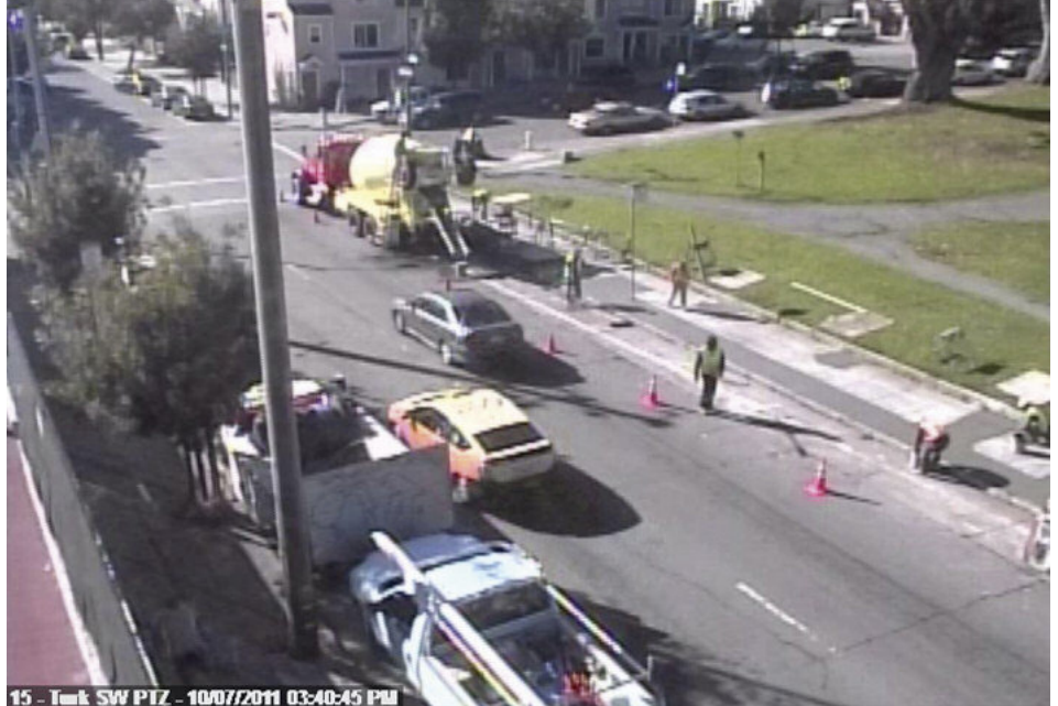
This frame-grab was taken from a security camera on a nearby building just seconds before impact.
